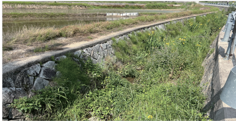
2018 Project Site – Sangchon Village Ditch
