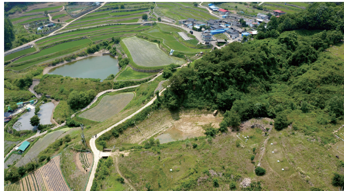
2022 Project Site – Gaho 2 Reservoir
